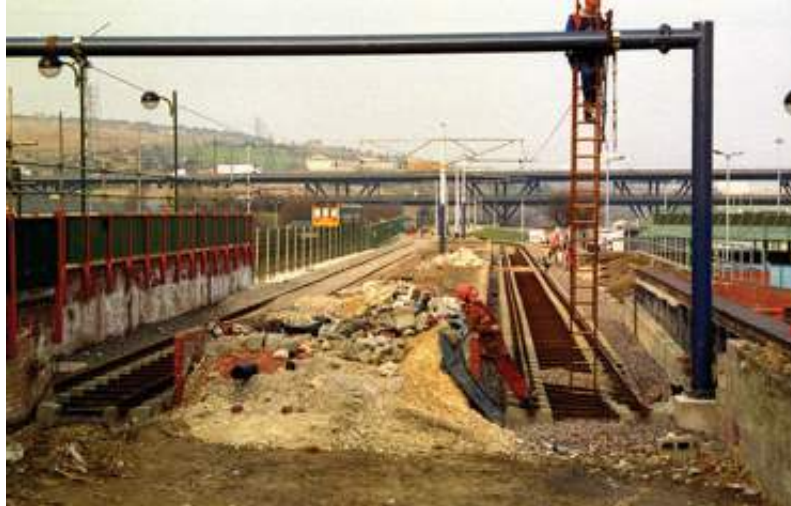
Figure 7: Installing a tram system in Edinburgh
